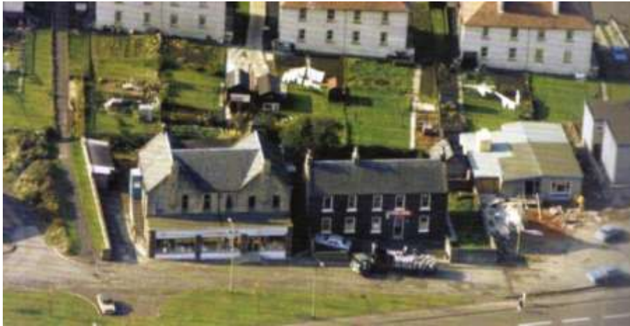
Illus 16: Left to right – Maddiston Co-op, Maddiston Inn, Salvation Army Hall. Note the re-alignment of the main road.
