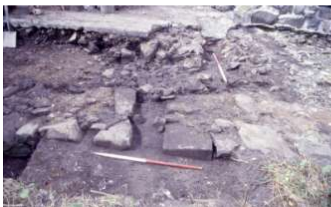
Illus 13: Drain in the east wall of Room 9, looking west, with late road metalling inside the room.
