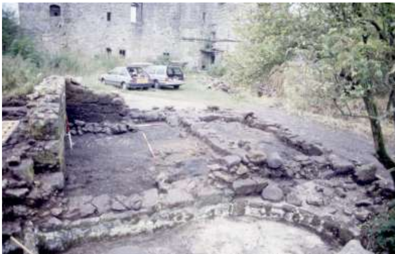
Illus 8: Room 5/6 looking SSW with the 1950s concrete duck pond in foreground.
