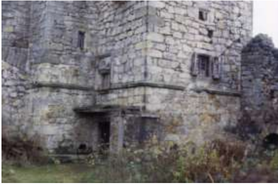
Illus 34: The foot of the tower with wooden shutters and porch still in place. The fireplace on the right is also a Miller feature.
