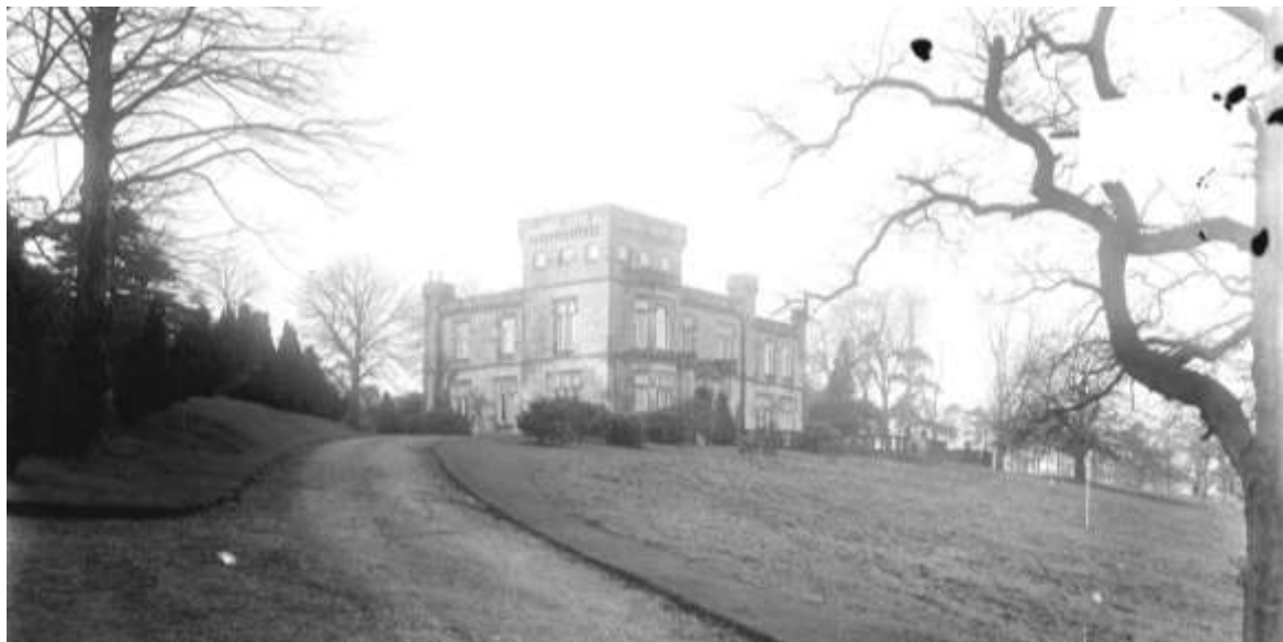
Illus 24: South Bantaskine House looking SW. The balustrade terrace can be seen on the right
