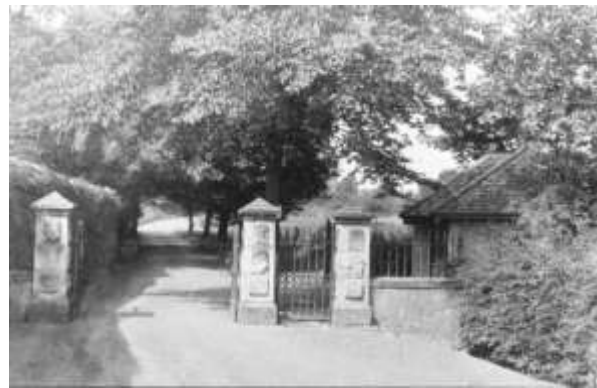
Illus 12 : The entrance gates and Well Lodge looking west up the East Avenue.
