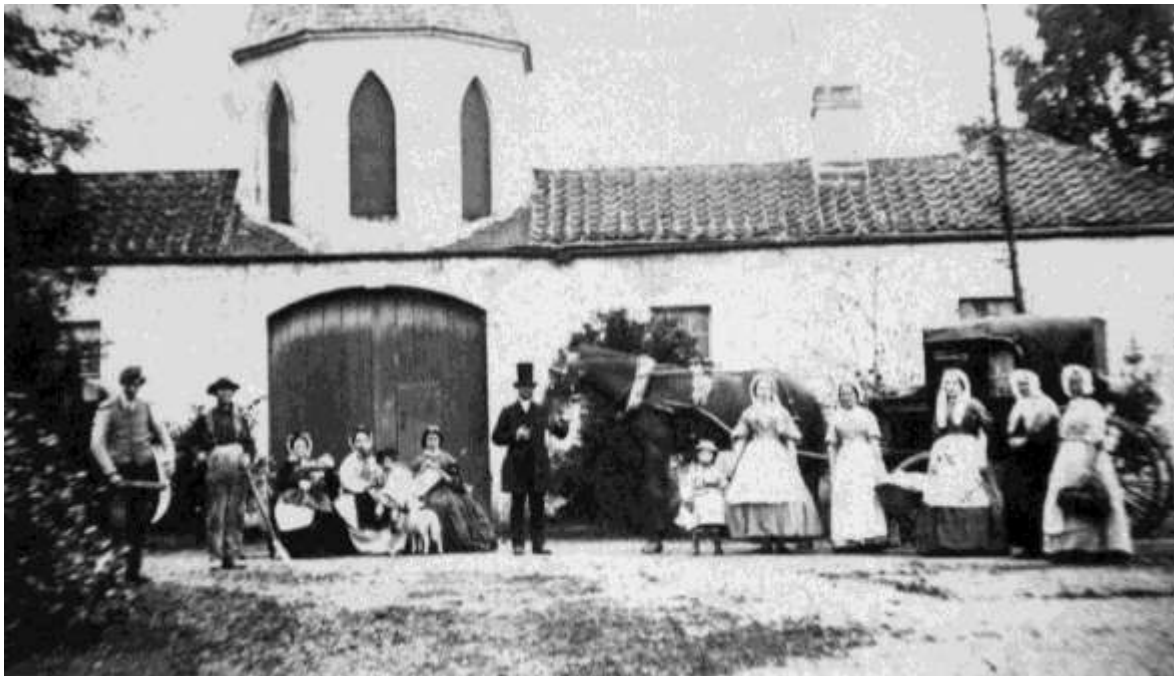
Illus 3: The court of offices or stable block looking south. The keystone over the arch and the plain Gothic style doocot show that this was an original feature of the 1807 complex.
