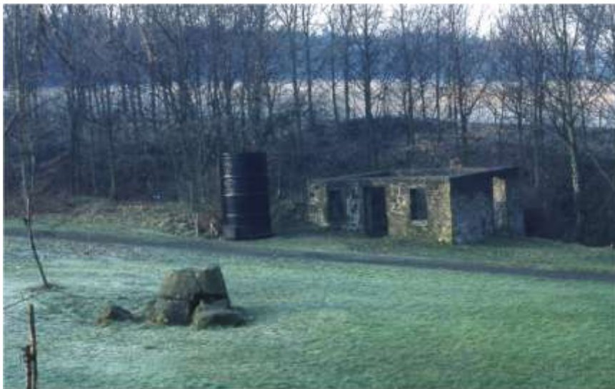
Illus 16: Watt's Workshop with the Schoolyard Pit cylinder to the left and fossil tree in the foreground.
