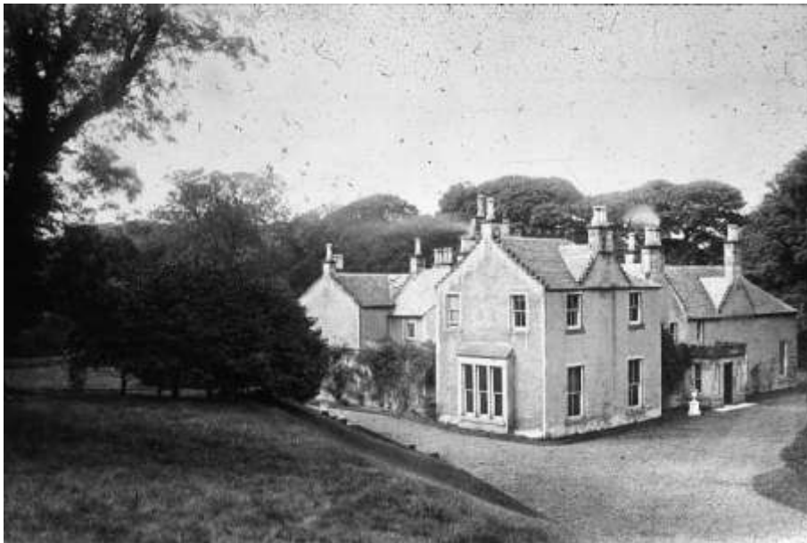
Illus 17: Dean House looking north-west.
