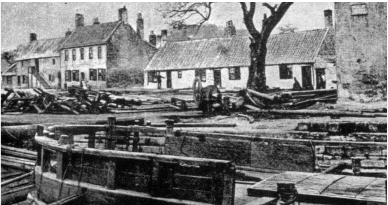
The Graving Dock at Carronshore
