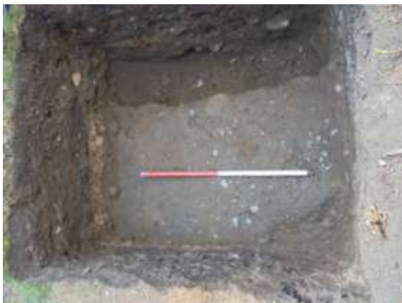
Illus 6: The surface of the upper road metalling in Trench B. The broken sandstone layer and the bituminous layer can be seen in section above it, with the sewer pipe trench at the top of the photograph.
