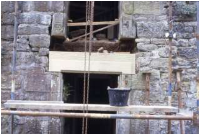
Illus: Replacing the lintels on the Callendar House Doocot.
